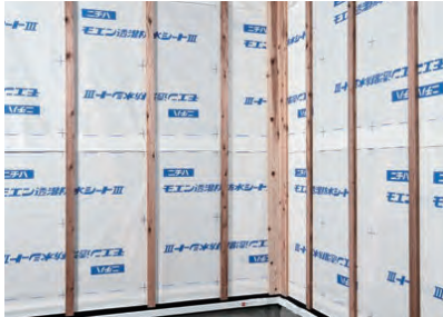
1. Installation of furring strips and building paper
