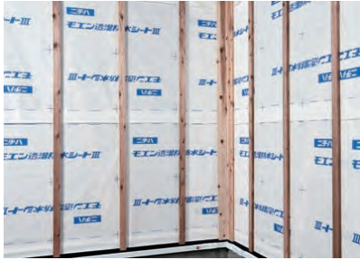
1. Installation of furring strips and building paper
