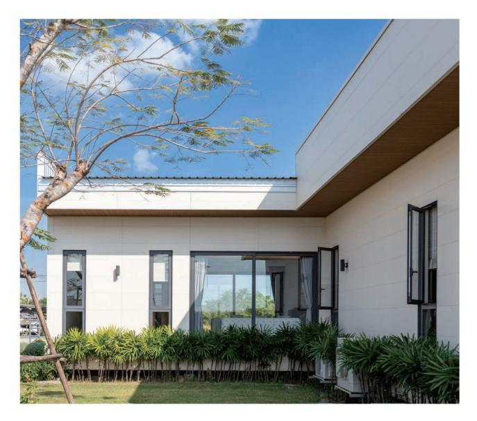
Four-side Tongue and Groove By using 1,820mm panels, it is possible to create a neat and beautiful wall surface with inconspicuous seams.
